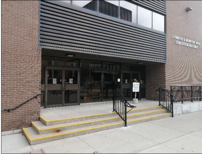
New handrails at front entrance, Education Building
