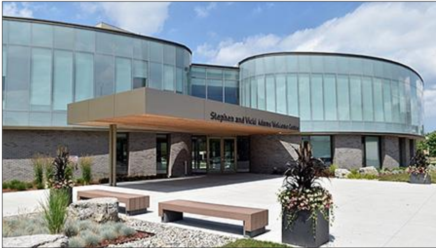
Exterior view of Welcome Centre Building
