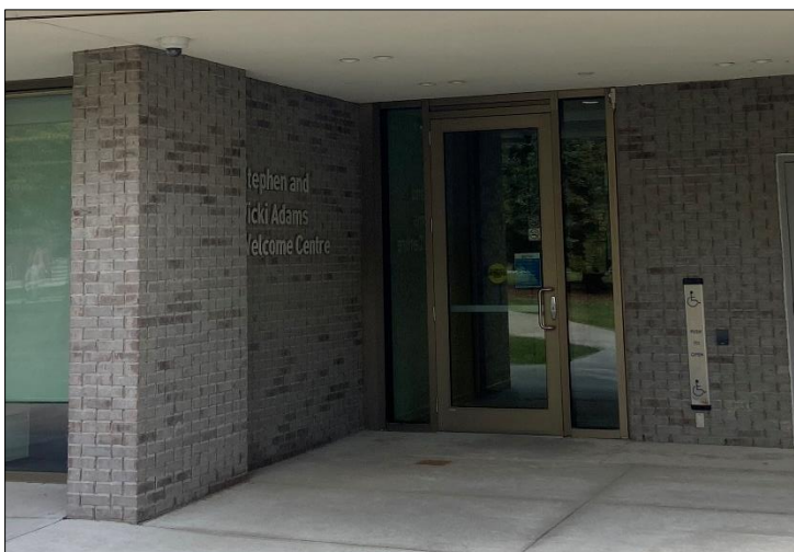
Accessible south entrance - ground level with actuators.
