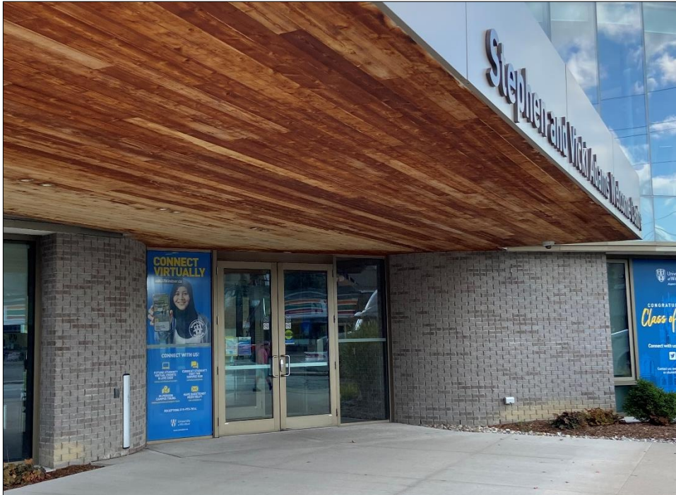
Main entrance to Stephen and Vicki Adams Welcome Centre. Ground level entrance with actuators.
