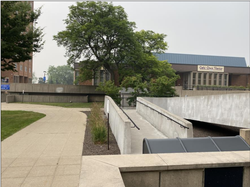
North side of Vanier Hall. Ramp to platform to the west provides access to main levels.
