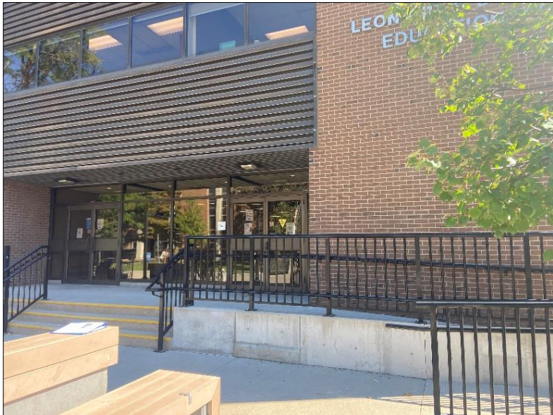
Main entrance to Leonard & Dorothy Neal Education Building with ramp and actuator.
