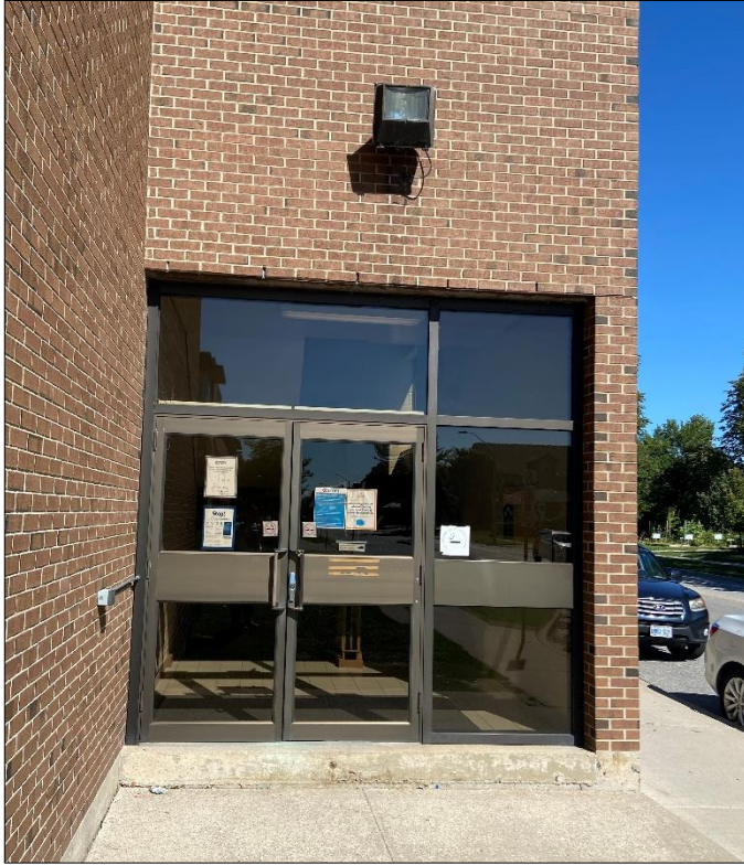
South Entrance with stair access.
