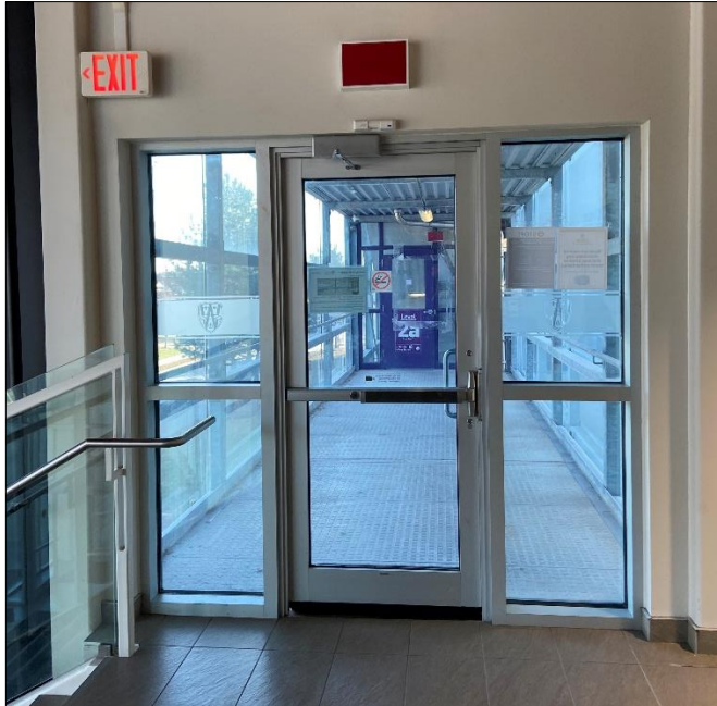
Entrance to pedestrian bridge leading to parking garage
