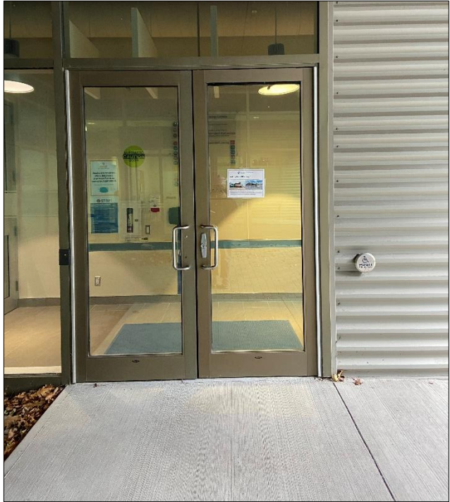
Exterior of entrance on south side of building
