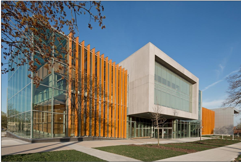
Exterior view of Ed Lumley Centre for Engineering Innovation
