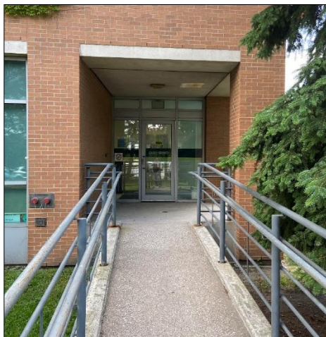
Northwest Entrance with ramp and actuator.
