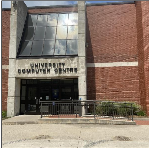
South entrance leading to University Computer Centre. Ramp and an actuator.
