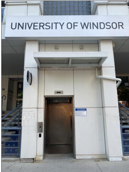
3 Elevator located on Ouellette Ave. to access 3rd and 4th floor.
