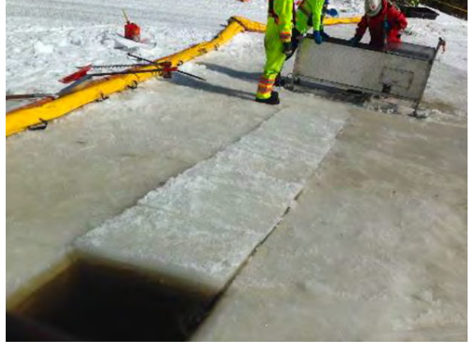
At left, an ice cutter chainsaw sled creating a space for oil to collect. At right, oil between the water and ice collects in the trench for easier clean-up. Source: ECRC, Cold Weather Training Document, provided to authors, 2023.
